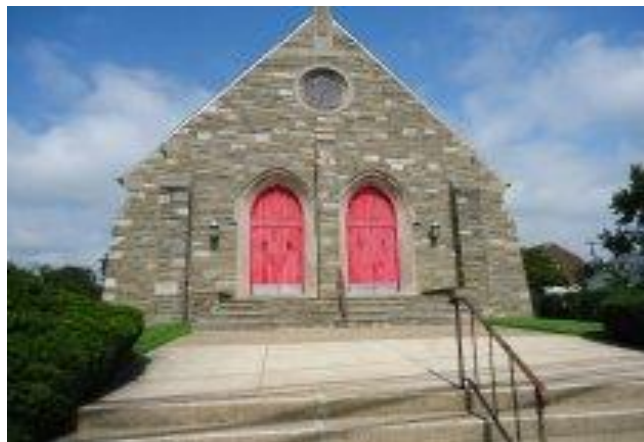
Sheep's Gate Presbyterian Church, Haverford Township Historical Society photo
