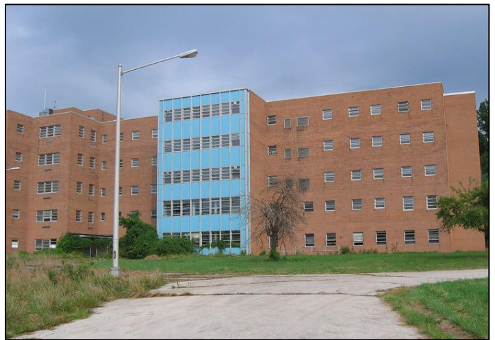
Photo of abandoned Haverford State Hospital – 2014
