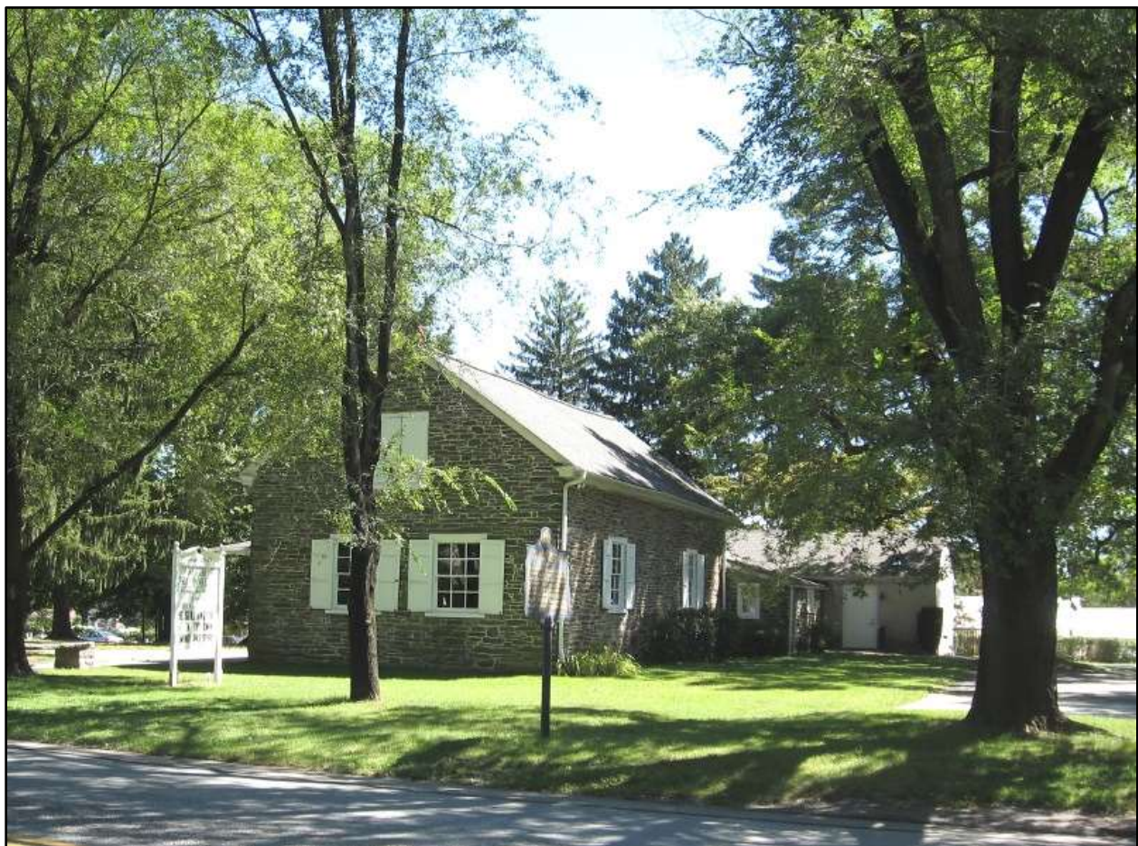
View from north of the Old Haverford Friends Meeting house, as it looks today from Eagle Road. (photo by author)
