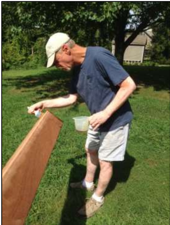
Jeff Wolfe making a new V-shaped wooden gutter for the rear of the Federal School.
