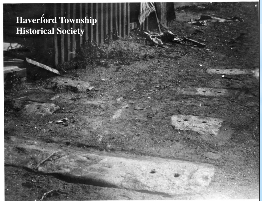
Primitive Railroad Stone "Sleepers"
