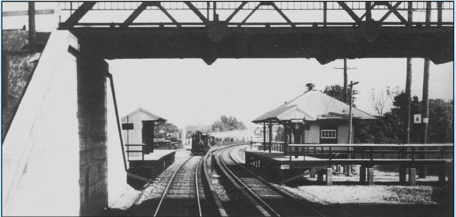
Rare view of original Haverford Station, with construction loco, 1908 (DeGraw Collection)
