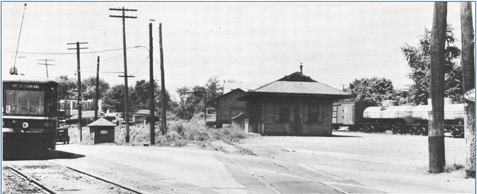
Llanerch Station and Freight House in 1938 (Collection of Harry P. Albrecht)
