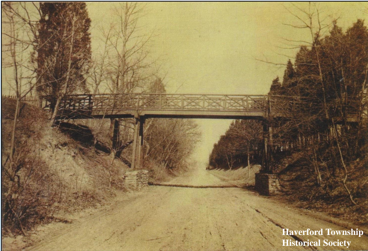
Old Meetinghouse Walk footbridge over Railroad Avenue (former railroad line)
