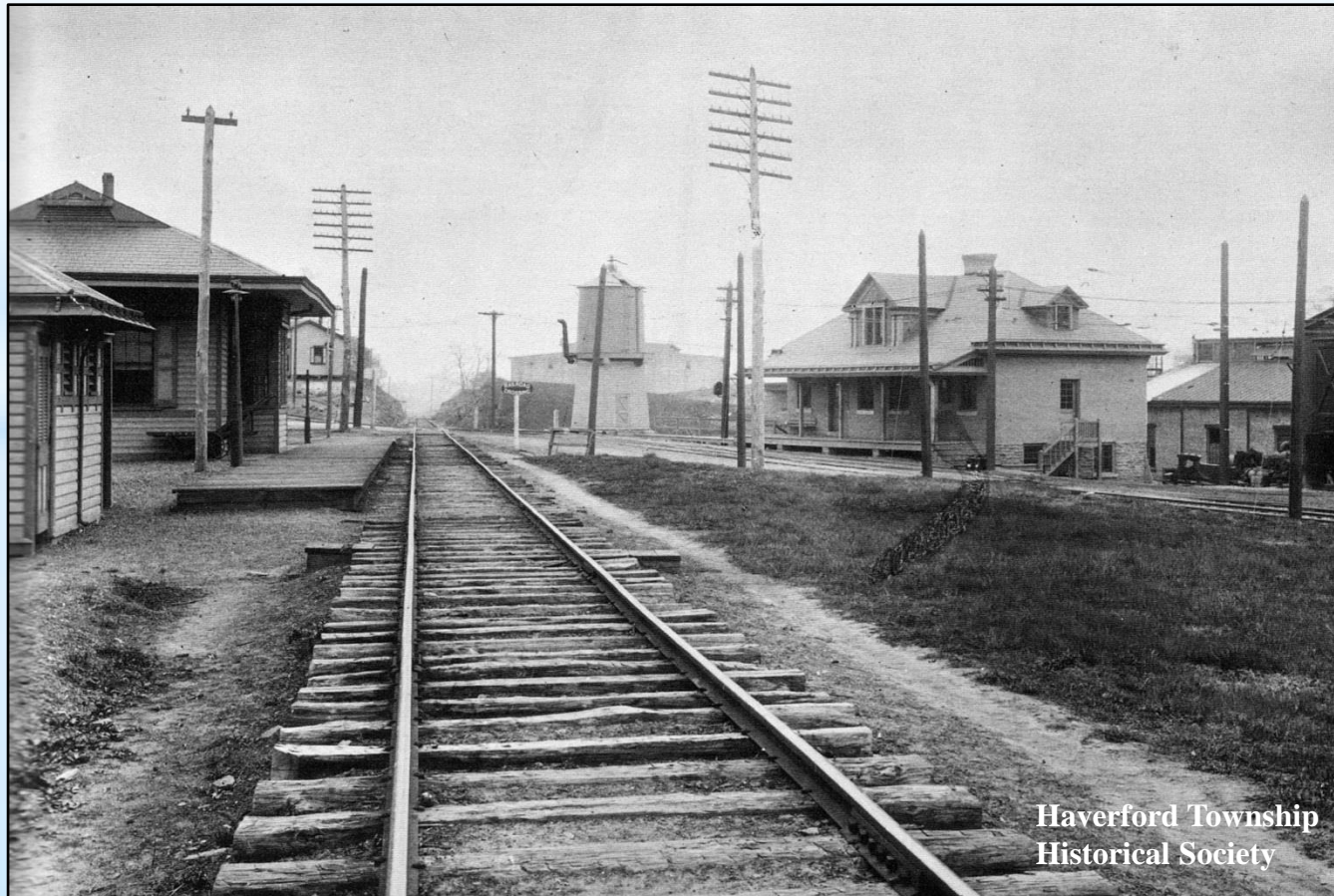
Llanerch Crossing looking southeast along Newtown Square Branch
