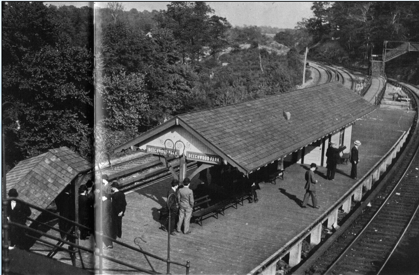
Beechwood Park Station, about 1907, with stairway to Brookline (DeGraw book)
